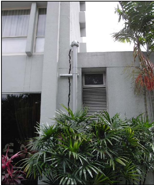
Annex structure on footings abutting buildings on piles
